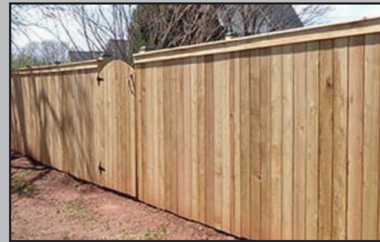
6' Tall Vertical Board with Cap and Trim
